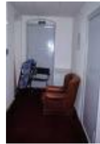
Obstructing an Exit
