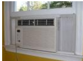
AC Window Unit
