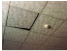
Moving Ceiling Tiles
